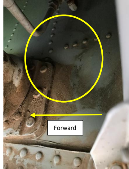
Zoomed in – deformation /buckling circled.
